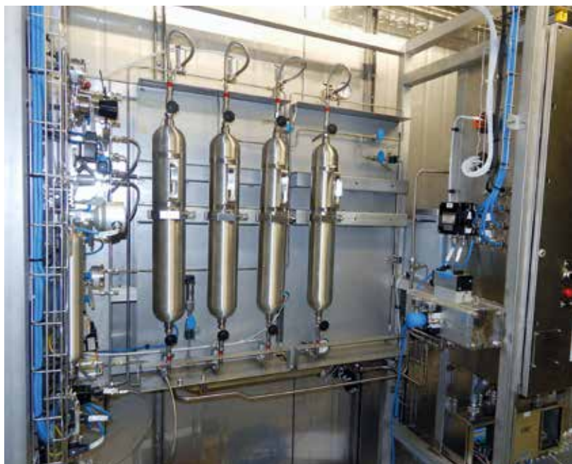
Typical Gas Sample Arrangement
